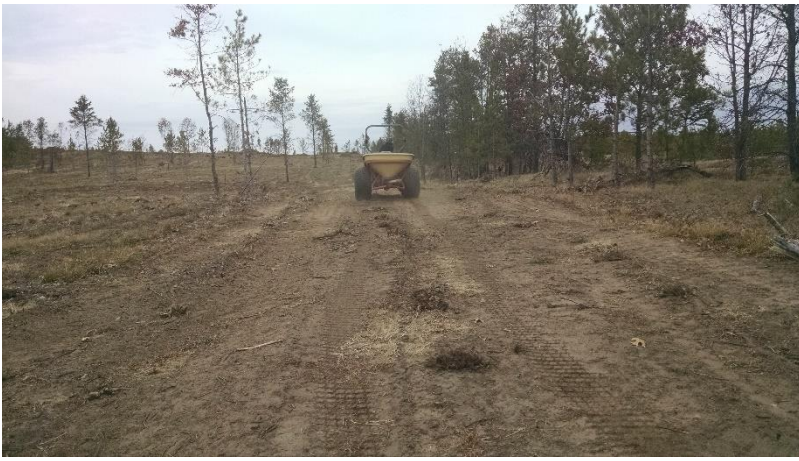
Seeding in fall 2014. To ensure proper seed distribution, seeding was done in two passes, one for small seed, and one for larger seed.
